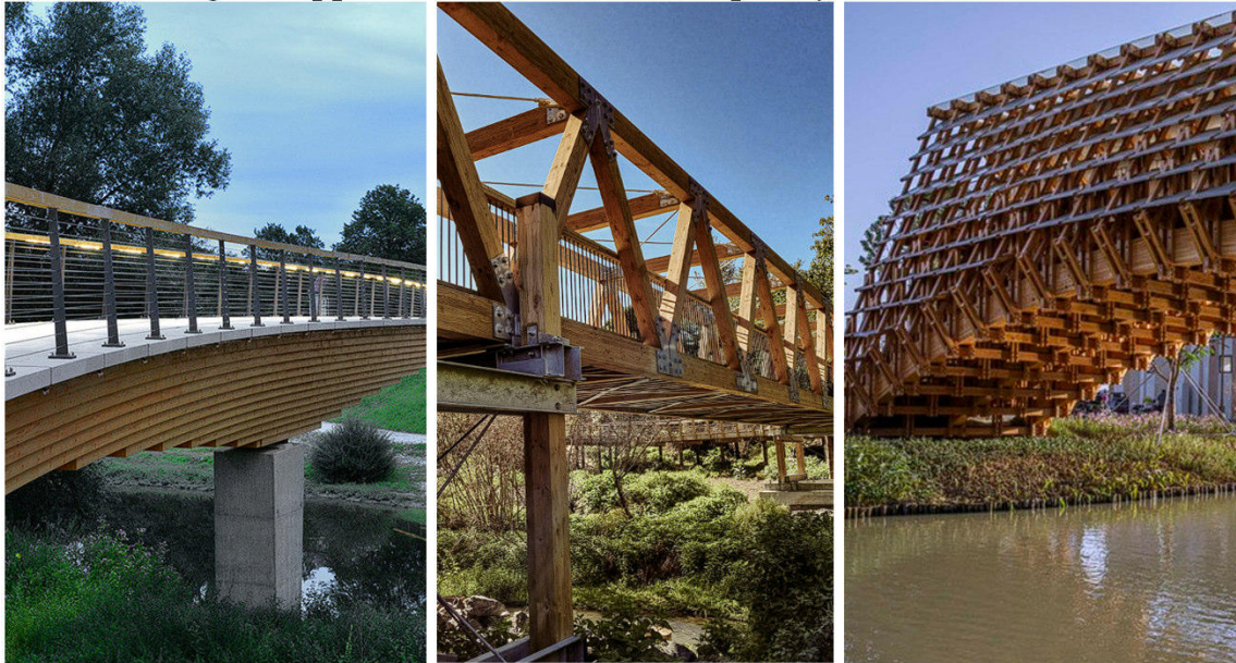
Fig. 5. Timber bridges of different functions
